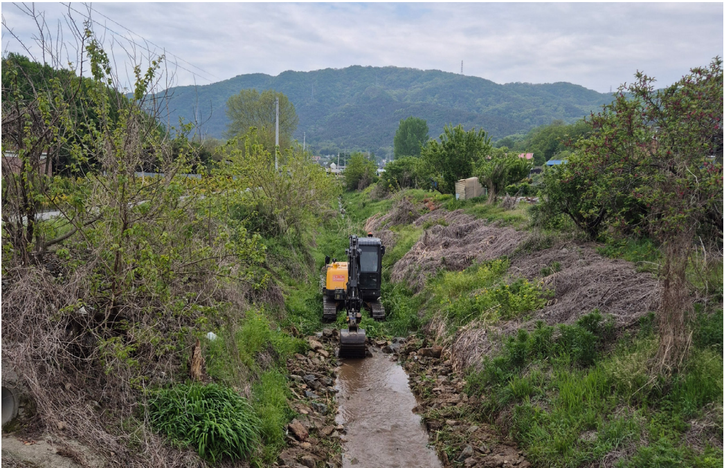
River Maintenance Project in Sindang Village
